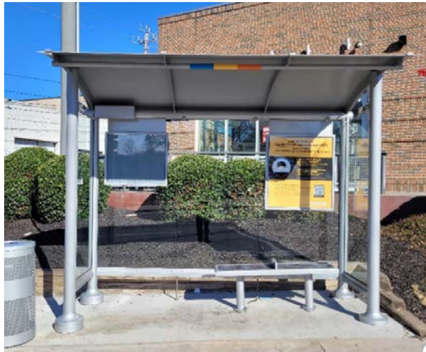
Newly installed bus shelters
